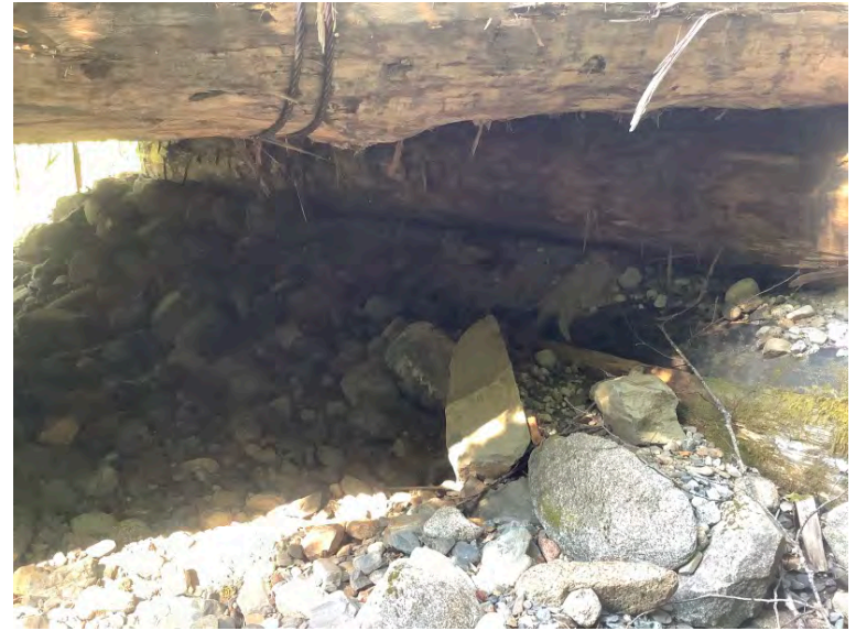
Right Bank Abutment when facing downstream
