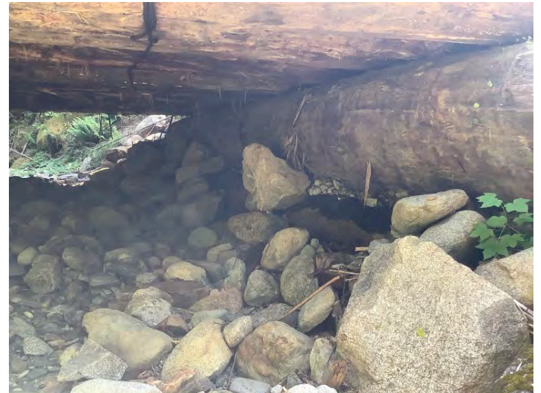
Left Bank Abutment when facing downstream
